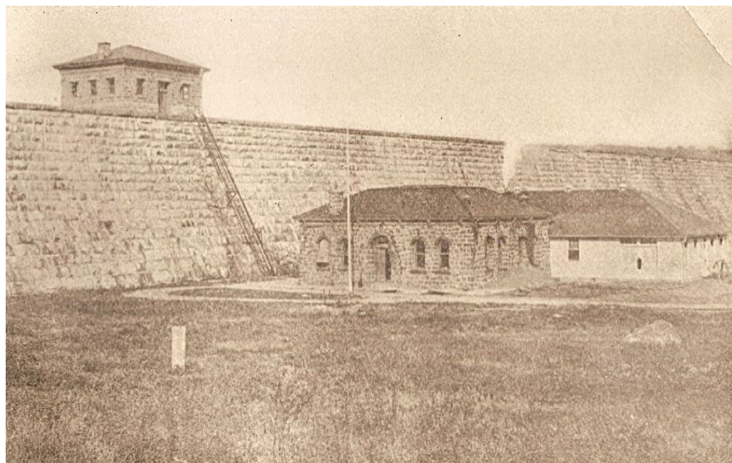
Boonton Reservoir – Chlorination Plant. 1909. Jersey City, NJ. waterandhealth.org
