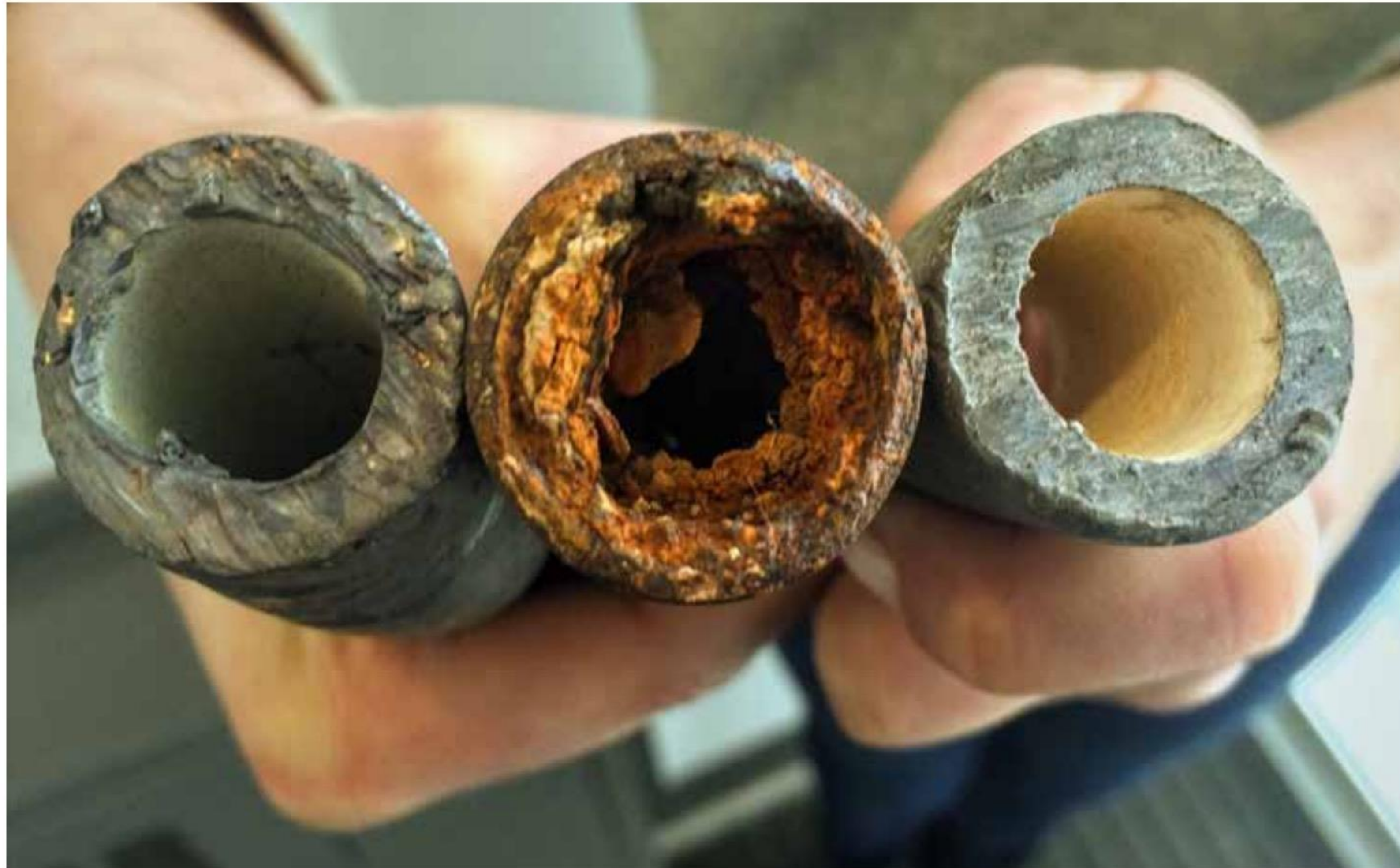
Pictured from left to right are a lead pipe, a corroded steel pipe, and a lead pipe treated with protective orthophosphate. Orthophosphate creates a film coating inside of lead pipes that can act as a barrier, reducing at least somewhat the amount of lead that gets into tap water.
