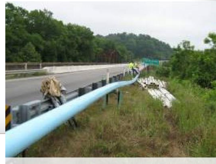
New pipe string installation
