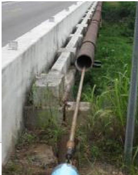
Pipe pull-in with pull rods
